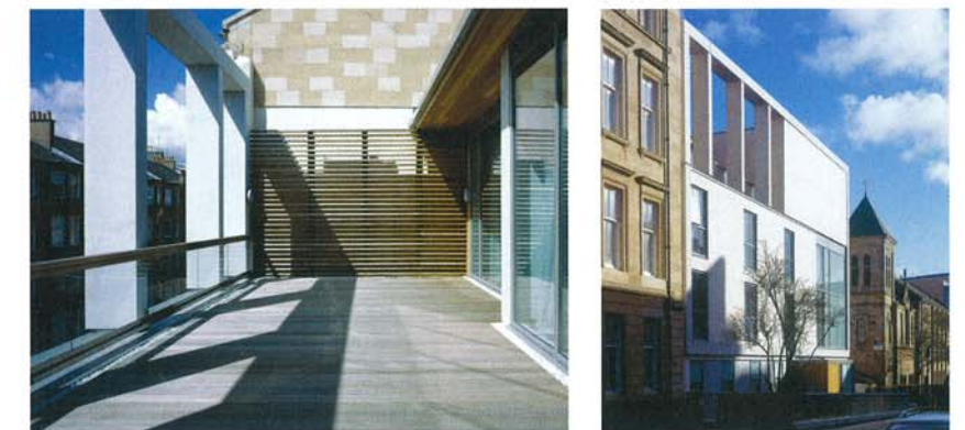
Top Main entrance to spirituality centre. Above Private roof terrace. Above right Oblique view to north-east. Plans Ground, first, second and third floors: 1 office, 2 residence reception hall, 3 group room, 4 interview rooms, 5 admin, 6 prayer, 7 team room, 8 entrance hall, 9 coffee, 10 conference, 11 bedroom, 12 parlour, 13 guest bedroom, 14 seating area, 15 laundry, 16 plant room, 17 kitchen and breakfast room, 18 dining room, 19 sacristy, 20 residence chapel, 21 timber deck, 22 superior's bedroom, 23 living zone, 24 tv room. The bedrooms are concealed from the main spaces and, as the priests' only private spaces, are generously sized. Internally, Elder & Cannon has attempted to create an interesting sequence of spaces which manage the priests' dual needs for privacy and welcome.
